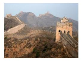
plants and loose bricks, you can still appreciate its astonishing beauty and impressive construction. The watchtowers were built to a range of designs giving each in turn a different look whilst the mountainous nature of the countryside required steeply rising and plunging parapets and other special features such as perpendicular obstacle walls to aid defence.
